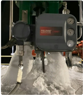
▲ Example of ice buildup on a critical control valve
